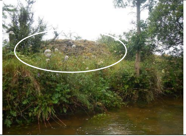
Figure 200: Gw 055. Heaps of spoil (white ellipse) previously dredged from the channel were a common occurrence along the river in adjacent fields.
