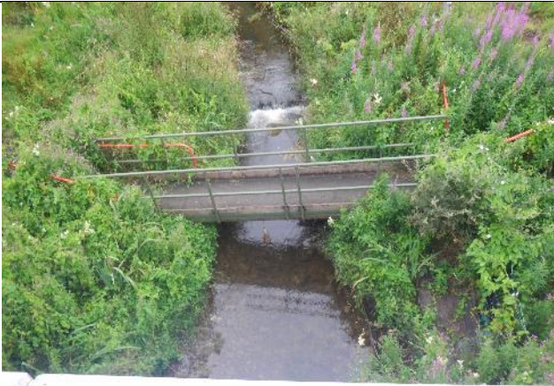
Figure 119: Sw 022 (53.956188, -8.990864). Further small weirs were observed from the new N26 road bridge. The geomorphology of the stream could be greatly improved by removing or at least notching the weirs. From the substrate observed it is likely that the river was capable of supporting large salmonid spawning and could be important for recruitment if naturalised.
