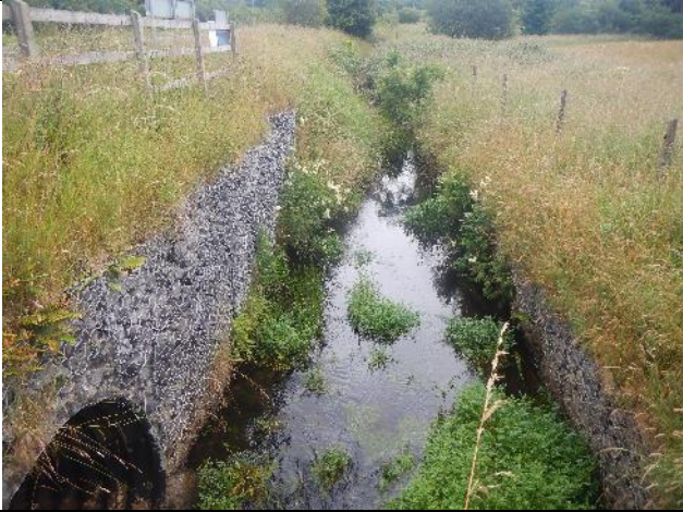
Figure 125: Sp 005 (53.927077, -8.95976). U/s of the N5, the watercourse was realigned, and armoured, but habitat quality was relatively good for a uniform channel, enhanced by vegetation.
