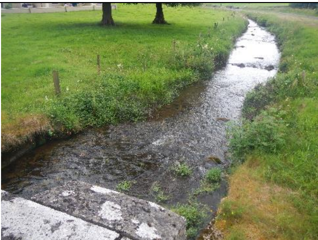
Figure 133: Sp 024 (53.935768, -9.016543). Although clearly dredged to a uniform capacity, habitat at the next location remained reasonably good for juvenile salmonids, particularly fry and 0+ parr, but lacked shade and cover. This area could be greatly enhanced with woody material/flow deflectors and a treelined strip.
