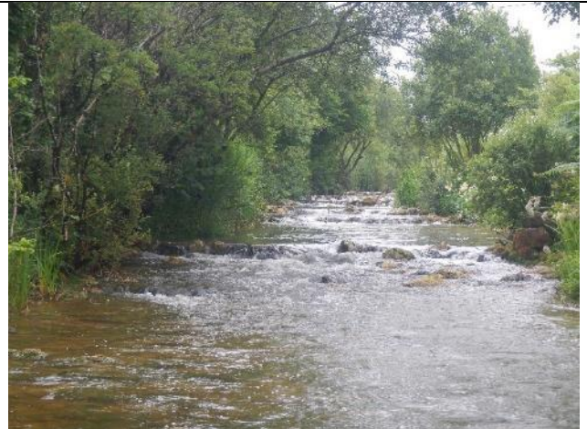
Figure 184: GI 089 (53.86989, -8.985915). Numerous weirs created (apparently relatively recently installed) pools in a long uniform section but, in conjunction with the long section of weirs u/s will have a significant detrimental impact upon sediment transport and habitat utilisation, forming behavioural and in some cases physical barriers.
