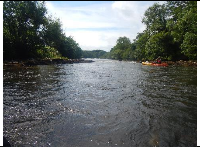
Figure 45: Mo 142 (53.94636, -9.044632). Paired groynes provide some flow deflection and acceleration but, ultimately, the habitat recovery of the river Moy would be better served by maintaining a channel free from man-made structures, that facilitates natural depositional features of coarse sediment, wherever the flow dictates (not artificial, static groynes).
