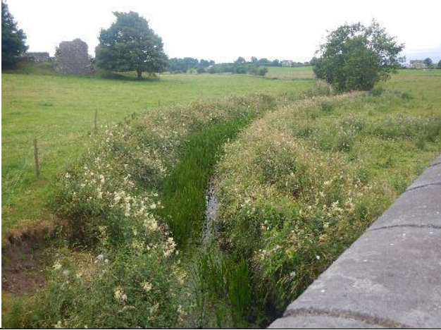
Figure 289: Ou 001 (53.935622, -9.105347). At the first spot-check, the Oughtagh River was uniform and over-capacity, with emergent vegetation encroaching into the channel. While this is a symptom of the issues, the channel narrowing was accelerating flow velocities and the watercourse would be expected to hold some juvenile trout.
