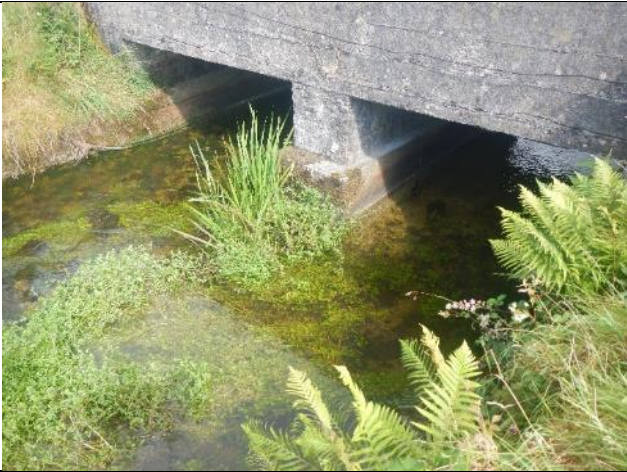
Figure 169: GI 046 (53.84461, -8.898523). The bridge crossing at the next spot-check posed no issues for fish passage and the slight narrowing and shade gave a glimpse of the higher quality habitat that could be achieved with a more naturally varied channel.
