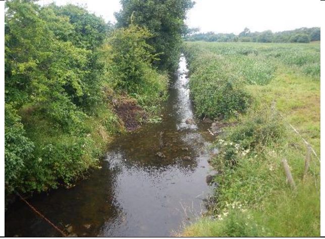
Figure 147: Ki 025 (53.928437, -9.022557). Uniform, straightened channel and livestock access and poaching d/s of the bridge (RB).
