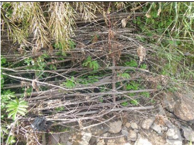
Figure 102: Mo 345 (53.949115, -9.12321). Bank erosion addressed with spilling. Rather than weaving the willow, it is usually beneficial to simply pin down a rough matrix of brash that traps fine sediment and create a growing medium. Horizontal spilling effectively hangs in the air, so will never grow, as the cross pieces receive no water or nutrient, and they create less roughness.
