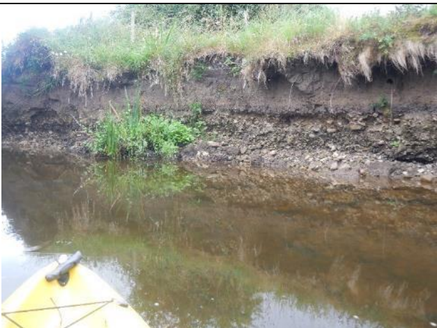
Figure 239: Gw 261. In some areas, slow, natural erosion should be seen as a positive process, providing additional coarse substrate to the river. This is in stark contrast to the exacerbated erosion around drinking bays and unfenced banks.
