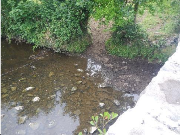
Figure 298: St 018 (53.915868, -9.132168). Significant poaching and fine sediment input were occurring at the L17141 road crossing. A long section u/s was inaccessible, in which water from the larger Little Strade River had bolstered the flow. Aerial photography shows past river channels in wet ground around 53.9025143, -9.1307923 may offer potential for restoration.
