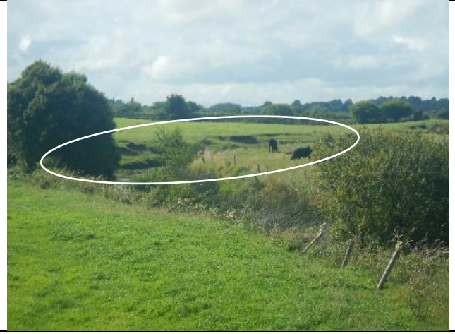
Figure 164: GI 031. Progressing d/s, the LB was unfenced and slumping (white ellipse).
