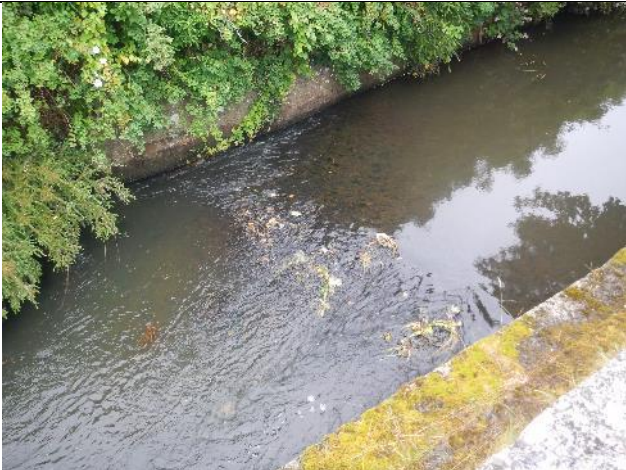
Figure 259: Tr 018. Occasional gravel bars had formed, demonstrating the requirement for width to facilitate coarse sediment retention, as well as narrower areas to create scour and depth. This demonstrates an issue with channel uniformity, rather than excess capacity. Increased flow sinuosity would facilitate more natural diagonal riffles that would better accommodate a range of flows.
