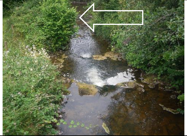
Figure 149: Ki 033. Three boulder weirs d/s of the road bridge. The Moy flows past right to left (white arrow). These still represent an obstruction in most flows but are an improvement over a much larger step. A continual rock ramp easement/bed regrade would be more in keeping with best practice, offering passage in a broader range of flows. This could unnecessarily delay fish entering the trib.
