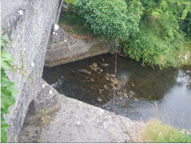
Figure 146: Ki 022 (53.928447, -9.022527). The road crossing/culvert was passable by fish.
