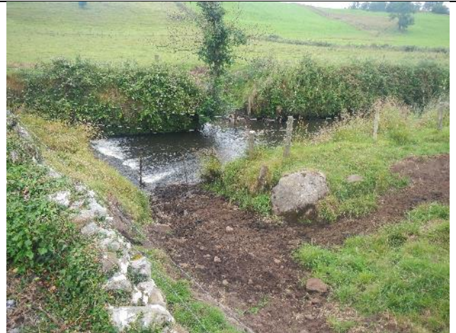
Figure 266: Tr 041 (53.866442, -8.891247). At the next spot-check d/s, significant poaching of cattle drinks at both bank sides created an issue. The perched bridge footings also created an obstruction which could be eased with baffles and/or a rock ramp d/s.
