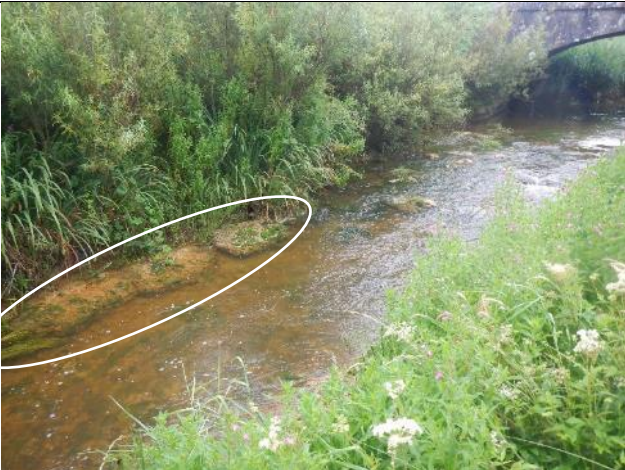
Figure 183: GI 077. From the R320 road, the Glore and then Gweestion were surveyed by kayak. Immediately d/s of the R320, in-channel habitat work had been undertaken, including stone groynes (white ellipse) and weirs.
