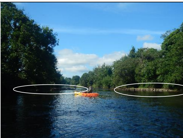
Figure 54: Mo 185 (53.934508, -9.050283). Where groynes are paired but slightly offset (white ellipses), they provide some more positive lateral flow deflection, but in most scenarios, it would still be preferable to simply allow natural depositional/gravel bed features to dictate the flow diversity.
