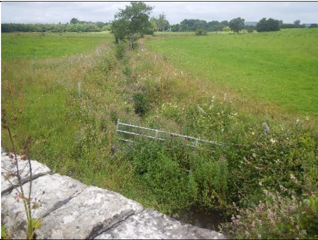
Figure 251: Gw(T3) 001. The third small tributary of the Gweestion that was inspected was of a similar character to the lower reaches of the second (Gw(T2)), being similarly straightened and set within the lower gradient areas of the valley. Again, emergent vegetation somewhat improved a uniform, over-capacity channel that really required major restoration.
