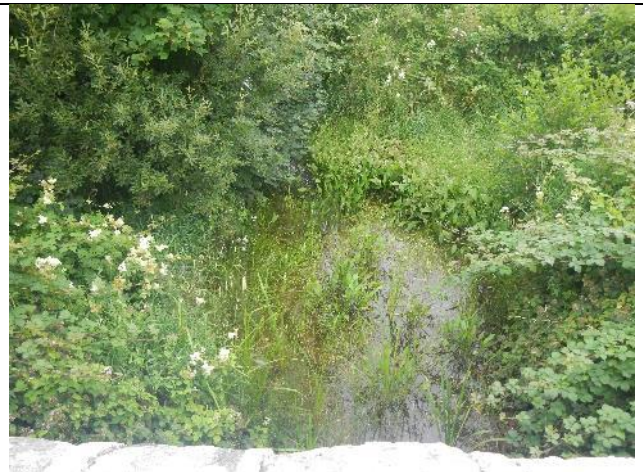
Figure 311: St(T2) 002. D/s of the road, the channel was weed-choked and barely discernible.
