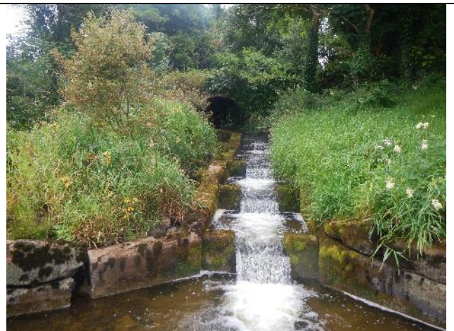
Figure 37: Mo 110 (53.944942, -9.033042). The second access to the Spaddagh is via an old-fashioned fish ladder. This will ease access, but the steps are larger than ideal for smaller fish and the pools are too small (~1.5m long is 50% of recommended) and shallow owing to sediment accumulation. The ideal solution would be to remove the disused bridge and footings u/s to reinstate free passage.
