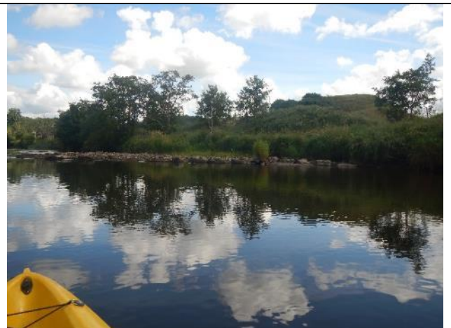
Figure 79: Mo 261 (53.931833, -9.088253). The largest groyne observed extended ~1/2 way across the channel and as with many others, will disrupt the natural transition of flow between two natural bends, but focussing flow hard along the LB after a large RH bend and before a LB bend.
