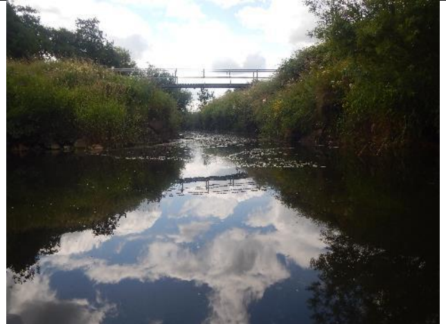
Figure 95: Mo 322 (53.93852, -9.11949). Although significantly realigned in its lower reaches, free access was possible to the Strade River, the size and substrate of which makes it a potentially important spawning tributary.
