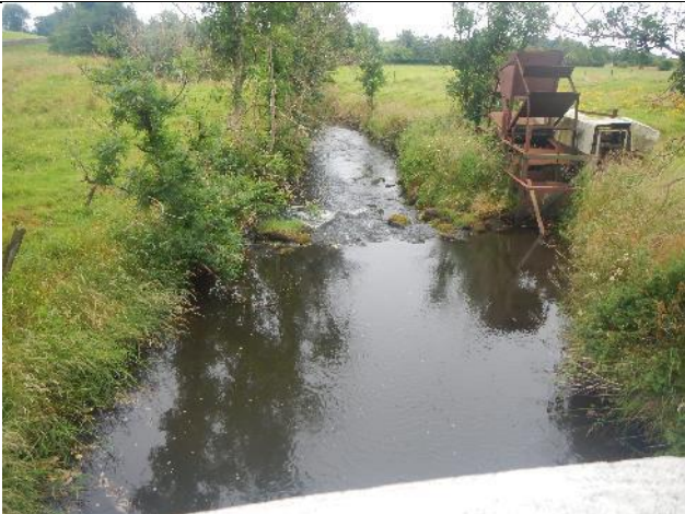
Figure 265: Tr 037 (53.865813, -8.88662). Signs of a small defunct hydropower installation, coupled with the mink trapping, suggests the landowner has an interest in the environment and may be open to river habitat improvements. Even removing the weir would be an improvement.
