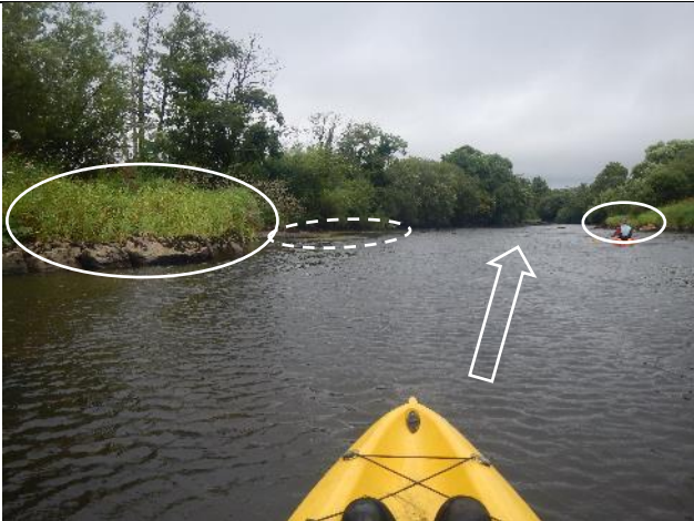
Figure 40: Mo 124 (53.94624, -9.03671). Poorly located groynes (white ellipses), focussing flow along a straighter course and detracting from the natural value of the bend. This was a common issue with many of the groynes, when the majority of flow should pass around the outside bend. The deflection had facilitated some gravel deposition d/s (dashed ellipse), but not in a useful or natural location.
