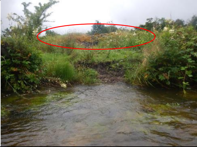
Figure 201: Gw 061 (53.881442, -9.00089). Drinking bay, bank erosion and associated inputs. Also note the dredged spoil in the background (red ellipse).
