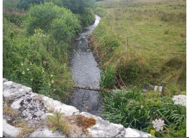
Figure 118: Sw 019 (53.949982, -8.973625). D/s of the Lagcurrach road bridge, a paired groyne and low-level weir were present just, with dredging having been undertaken recently, possibly because of sediment accumulation from the weir. The weir and at least LB groyne should be removed and drinking bay replaced with a pasture pump. Preventing further dredging would be highly beneficial.
