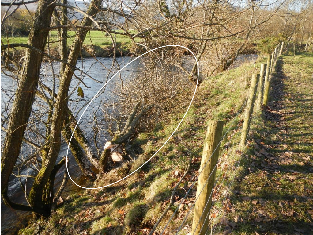
Figure 7. Willow trunks hinged into the river channel during a WTT habitat workshop, to provide low cover and structure. Numerous juvenile salmonids were subsequently observed sheltering in and around the new habitat.
