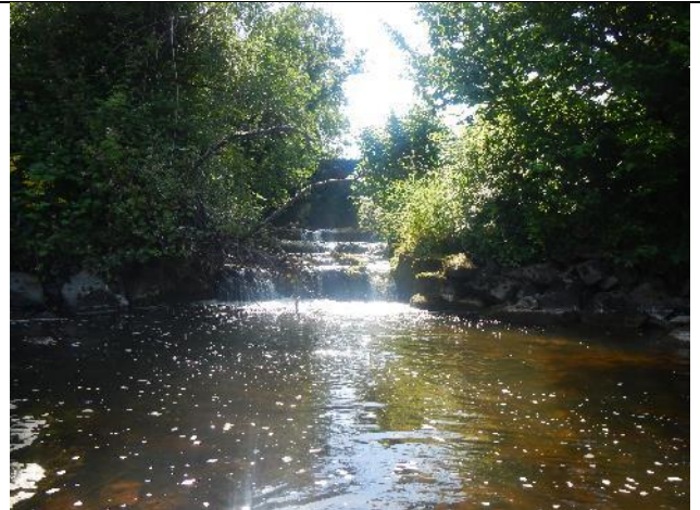
Figure 53: Mo 182 (53.934547, -9.050158). Access from the Moy to the Killeen River is inhibited by a series of boulder weirs. It was not evident whether these were scour protection for the bridge footings u/s or an attempt to ease fish passage over the footings, but access remains restricted.
