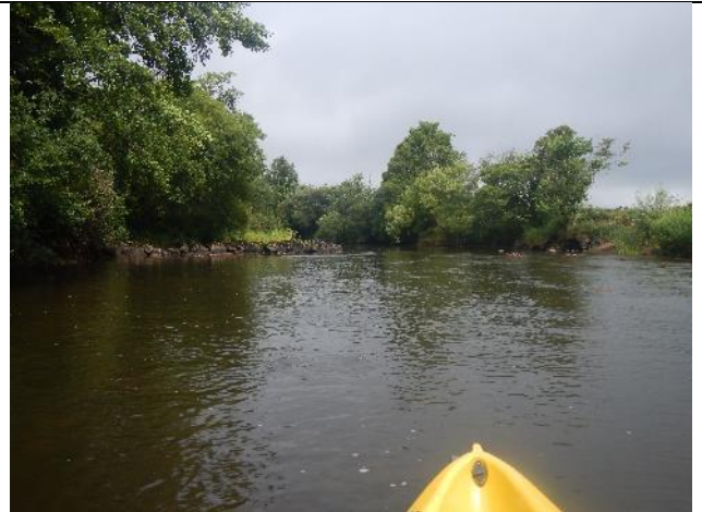
Figure 41: Mo 127 (53.946995, -9.0372). One of the 'better' placed groynes, on an inside bend. These were probably installed when the channel was significantly uniform and degraded post-dredging and benefits to channel morphology where probably achieved, but longer-term, it would be beneficial to remove them allowing more natural features to develop - which these groynes inhibit.
