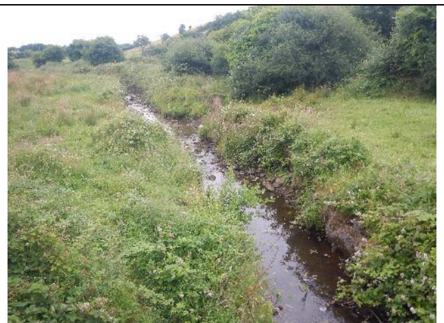
Figure 297: St 016 (53.893105, -9.132817). D/s of the Old Road, the river remained straightened and lacked buffer fencing, but the banks appeared to be reasonably well vegetated, apart from at crossing points. Fencing would be beneficial and restoration could be a possibility within the unimproved grassland.
