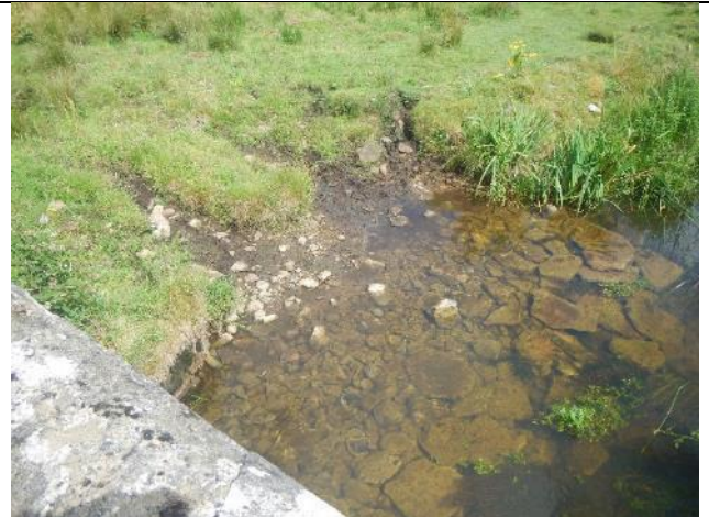
Figure 178: GI 067 (53.855302, -8.952265). Livestock poaching at a drinking point. Much of this area was protected by high, steep banks and/or buffer fencing, but some conspicuously weren't. The placement of stone within the channel does little to mitigate the issue.
