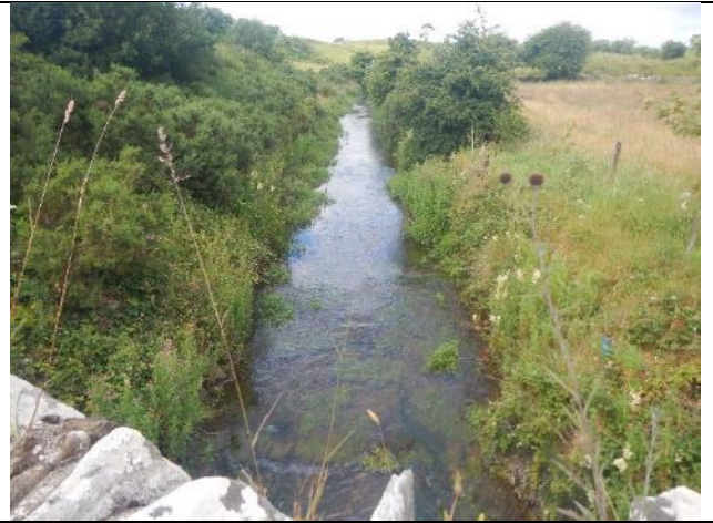
Figure 172: GI 0051 (53.851462, -8.927617). These straightened sections could be greatly enhanced by restoration/re-meandering or, at the very least, increasing variability in flow diversity and channel width with woody material.
