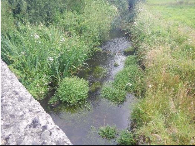
Figure 131: Sp 019. D/s of the bridge, emergent vegetation enhanced the habitat for fish and invertebrates. The bridge structure was passable by fish. Again, the uniform channel could be enhanced by installing habitat features.
