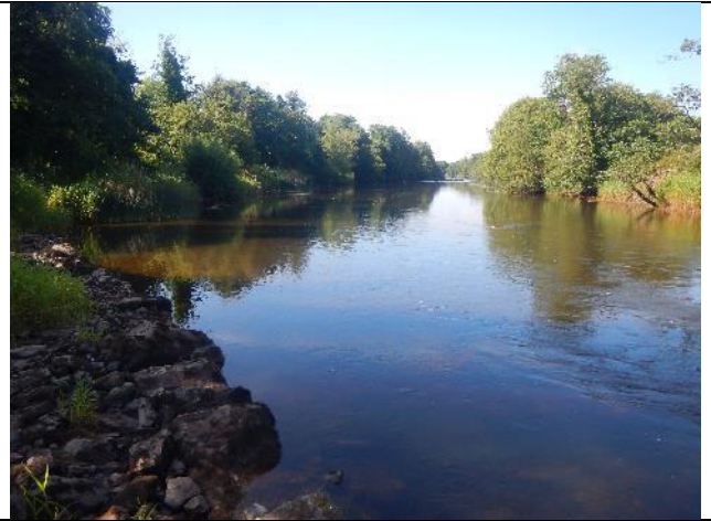
Figure 51: Mo 173 (53.937012, -9.047843). Flow was again encouraged to cut the corner d/s owing to the groynes.
