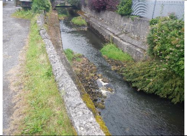
Figure 258: Tr 016. Habitat work immediately d/s: but as with many of the groynes on the Moy catchment, some were paired, reducing their benefit by unnecessarily constraining flow to the centre of the channel, rather than promoting sinuosity; they are also too closely spaced longitudinally. In this highly modified channel, they are an improvement, but the impact could be far more positive.
