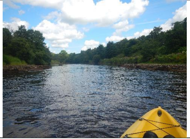
Figure 81: Mo 268 (53.935097, -9.087385). Paired groynes u/s of a single groyne on the inside bend (LB). The single groyne does push flow towards the outside bend, but the paired groynes u/s focus flow to the centre of the channel, inhibiting a more sinuous flow pathway down the channel.
