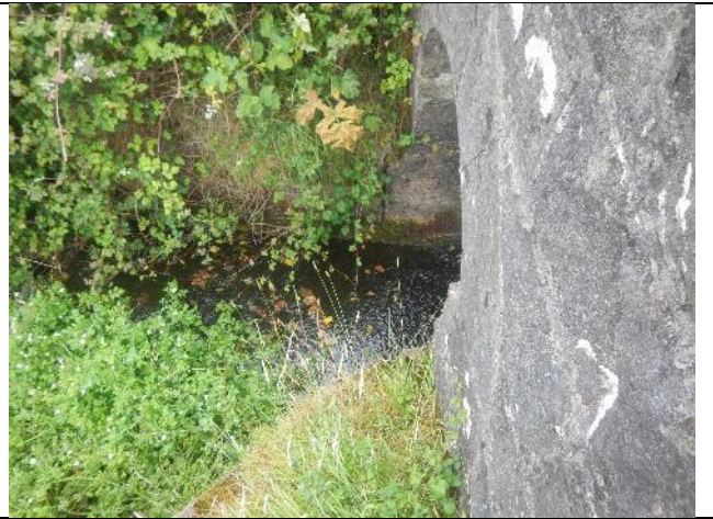
Figure 252: Gw(T3) 002 (53.916445, -9.054422). The tributary appeared to be accessible from the main river at the points observed, although shallow water over a smooth (presumed to be concrete) bed created a small obstruction at one of the road crossings.
